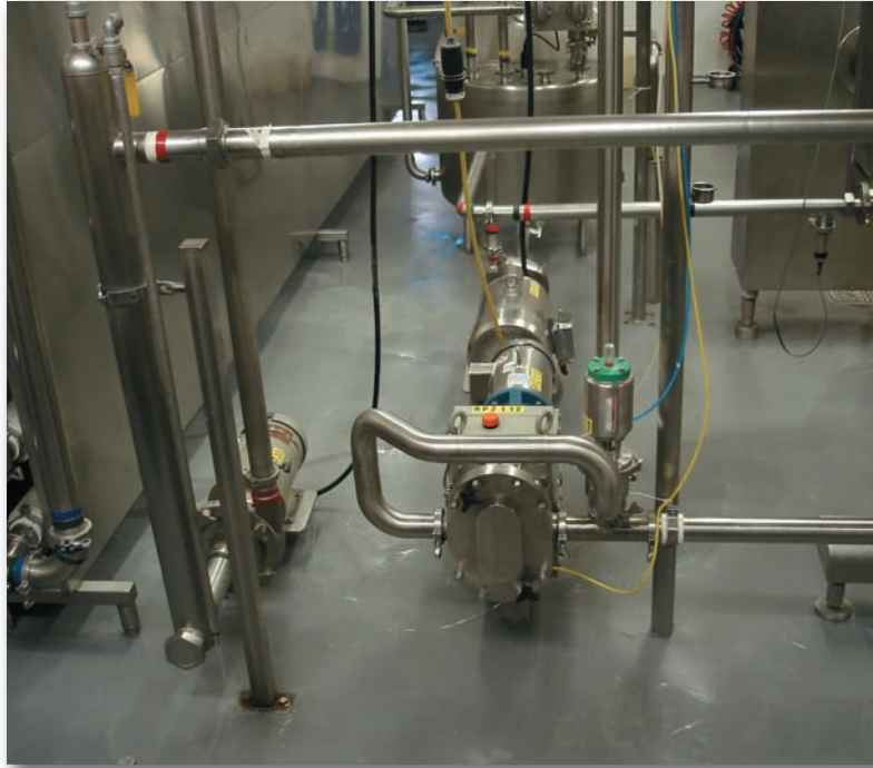
The Fristam FKL Positive Displacement pump reduces maintenance costs and downtime at Oskaloosa Food Products.
